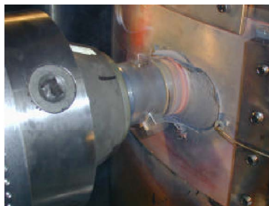
The early stages of a Cu canister weld. Note that the tool is operating at red heat
