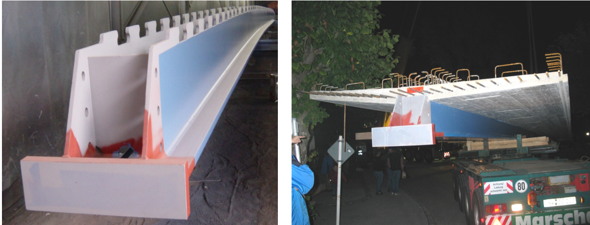
Fig. 8: Double-T arrangement for prefabricated composite bridge element
