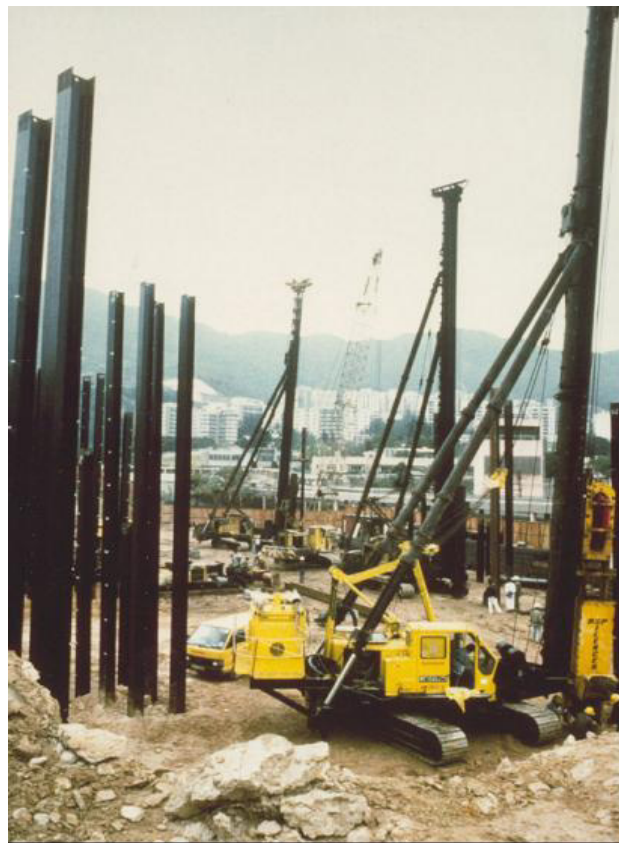
Fig. 4: Driving of HISTAR bearing piles in Hong Kong
