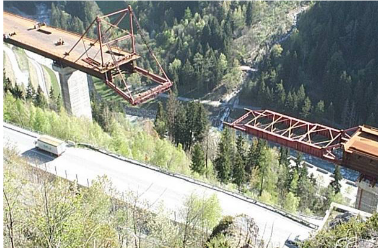
Fig.11 Connection of the bridge parts, built in two different yards (Aosta and Mont Blanc sides)
