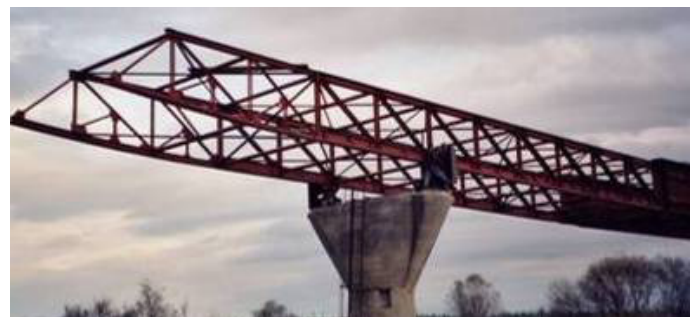
Fig.3 Arno viaduct (2001). Launching phase
