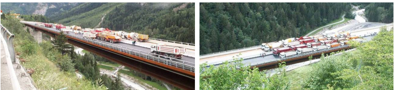
Fig.15 Final test of the Verrand viaduct
