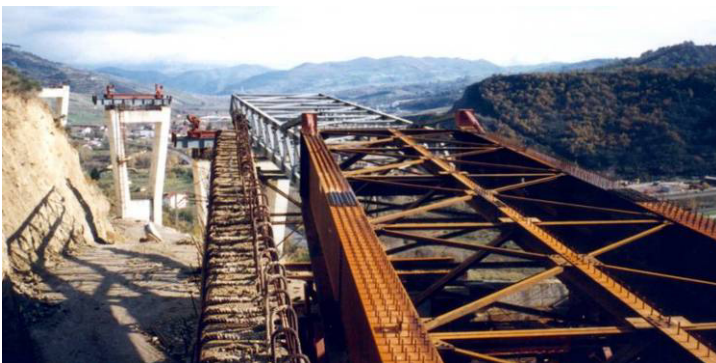
Fig.4 Calitri viaduct (2000). Launching phase
