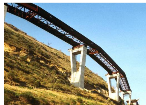
Fig.4 Calitri viaduct (2000). Launching phase
