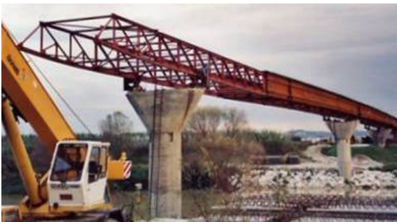
Fig.3 Arno viaduct (2001). Launching phase
