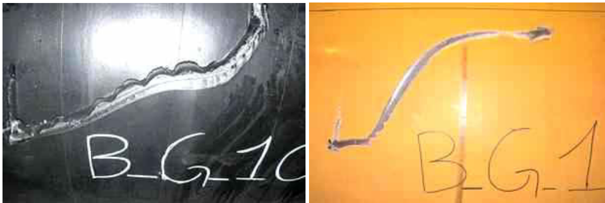
Figure 3 - Example of third party damages realized on line B coated pipes (FBE coated pipe on the left and HDPE coated pipe on the right).
