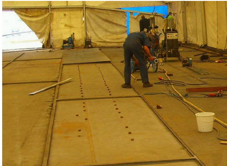
Figure 34: SPS-Overlay-technique to refurbish the steel deck of the Schönwasserpark-bridge Krefeld, Germany [Krupp]
