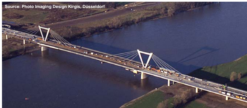
Figure 31: Rhine bridge Düsseldorf-Ilverich with tension tie in the pylons made of S460 TM [4]
