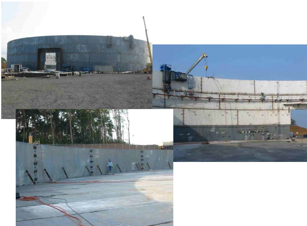
Fig. 9: Construction of flat bottom tank (capacity 132.000 m 3 ), Bioko Island/Equatorial Guinea
