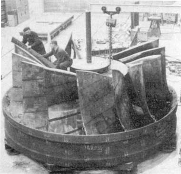
Figure 4. Assembly of a 67 tonnes Francis turbine runner in 1957. Manual metal arc welding with ESAB OK R6 consumables was used for buttering of joint faces and for final assembly welding (15).
