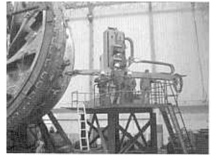
Figure 5. Mechanised SAW welding of Francis turbine runners for the Chinese Three Gorges hydro-power project [16].
