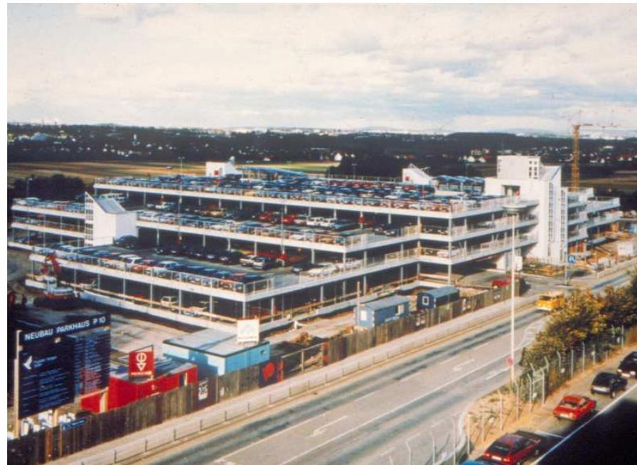
**Long span : no internal columns**
