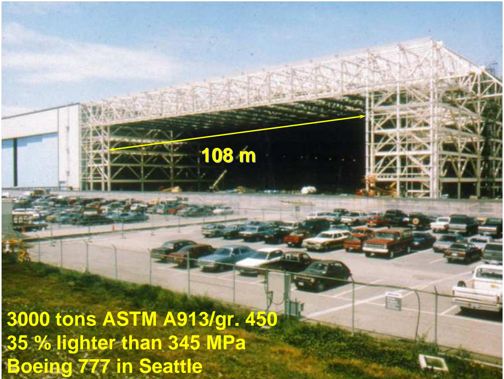
**3000 tons ASTM A913/gr. 450**
