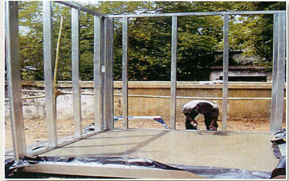
Frame of the small scale prototype building in construction
