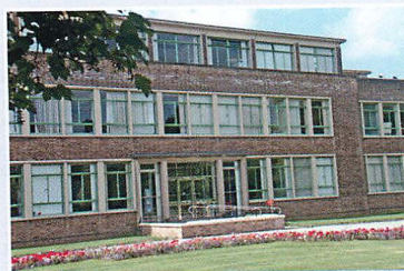
Swinden Technology Center
