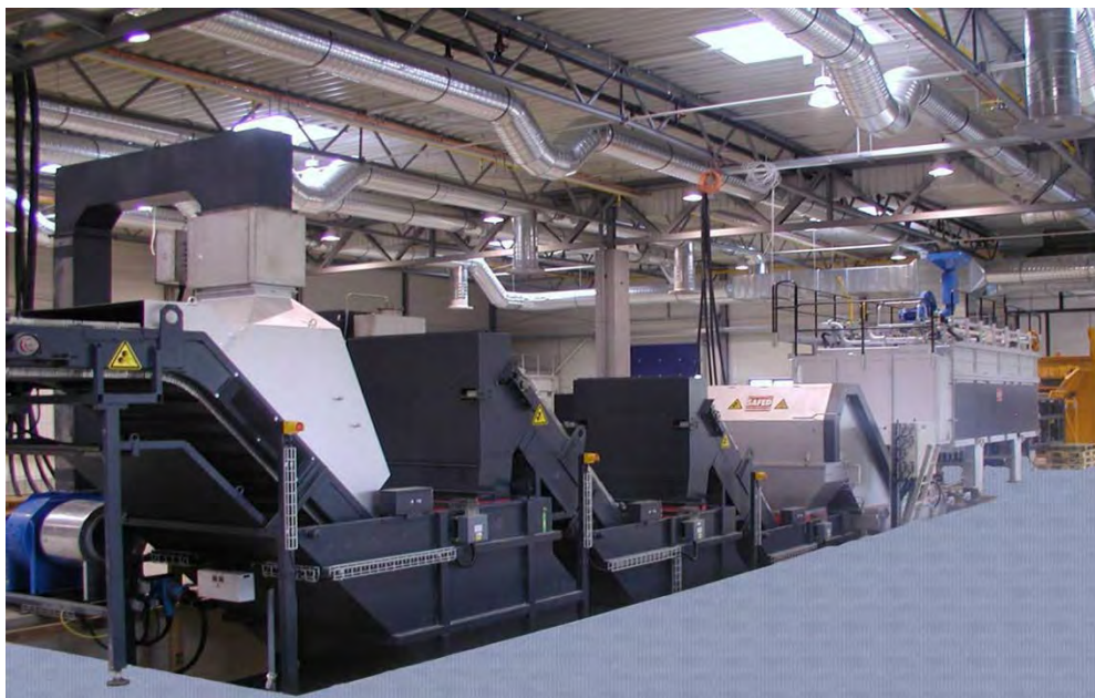
Figure 8: Conveyor belt furnace with salt bath and washers
